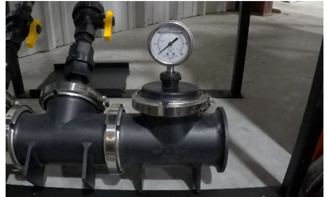
Dura Auto-Batch™ Direct Injection 3” Gauge Assembly
