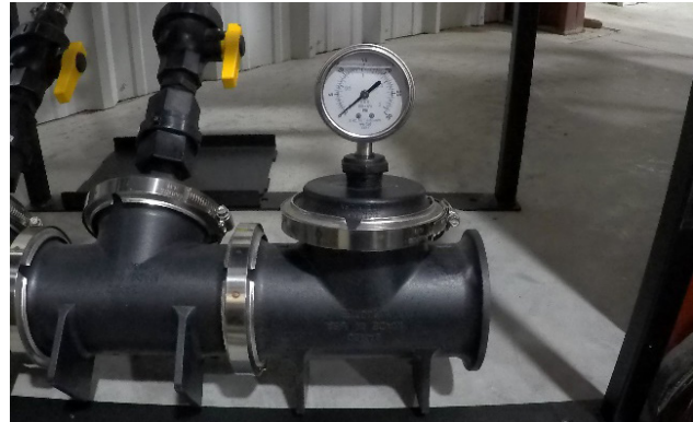
Dura Auto-Batch™ Direct Injection 3” Gauge Assembly
